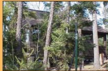
This cabin on Seagull Lake was protected by its working sprinkler system during the May 2007 wildfire. The cabins on both sides of this cabin did not have sprinkler systems and were destroyed in the fire.
